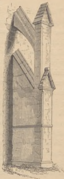
Flying Buttress, Hartlepool, Durham, c. 1220.
