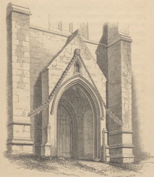
Porch, Rushden, Northamptonshire, c. 1300.
