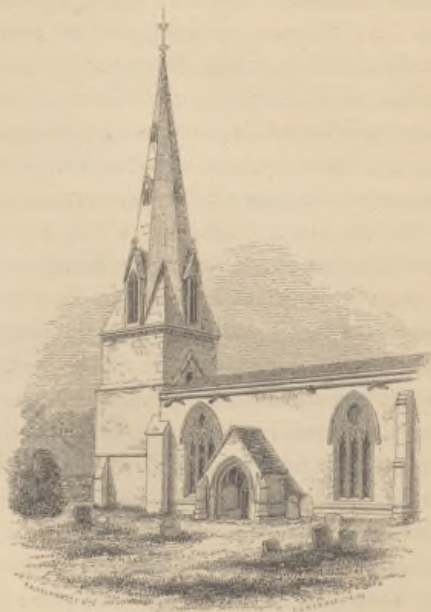
Spire of Ringstead Church, Northamptonshire c. 1200
