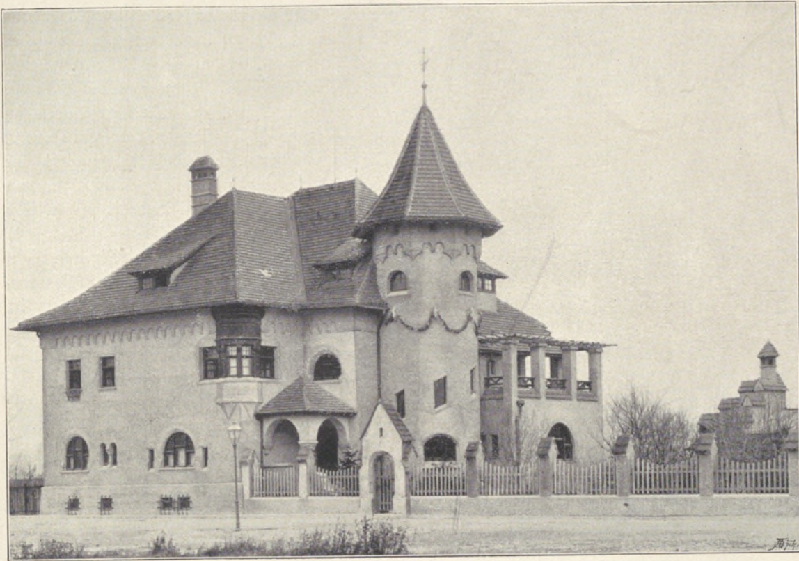
VILLA OBRIST A MUNICH
